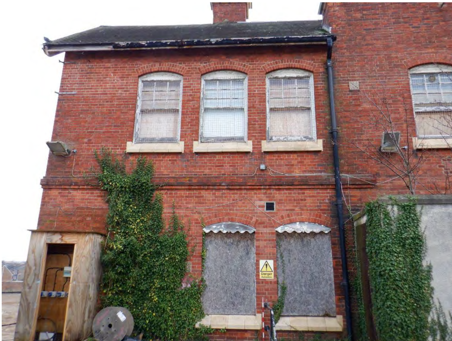
Plate 38: Window detail western elevation of office (December 2020)
