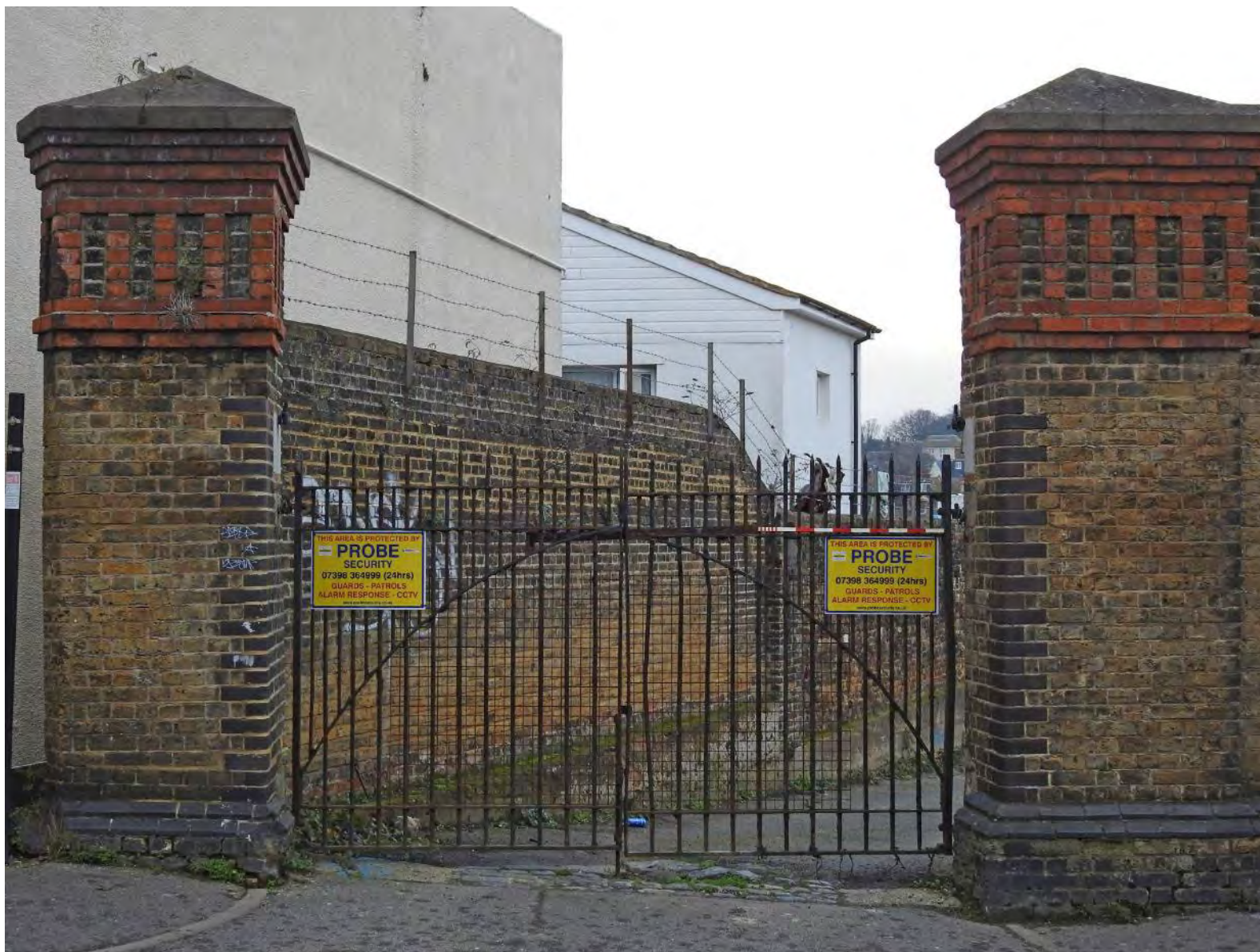
Plate 44: View of the south western gate (August 2021)
