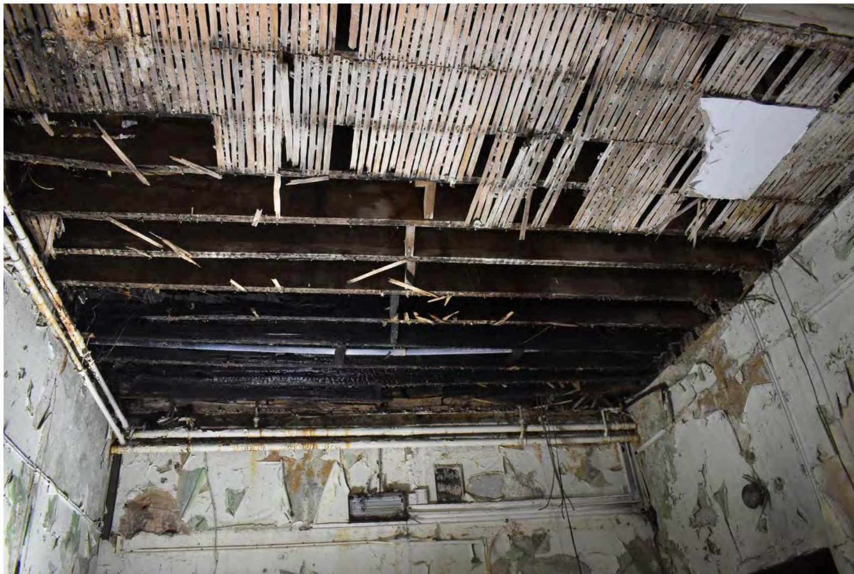
Plate 137: Main Office, Basement, Room C ceiling
