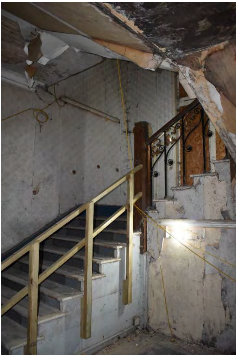
Plate 142: Main Office, Ground Floor, Room 1 Staircase (facing SE)
