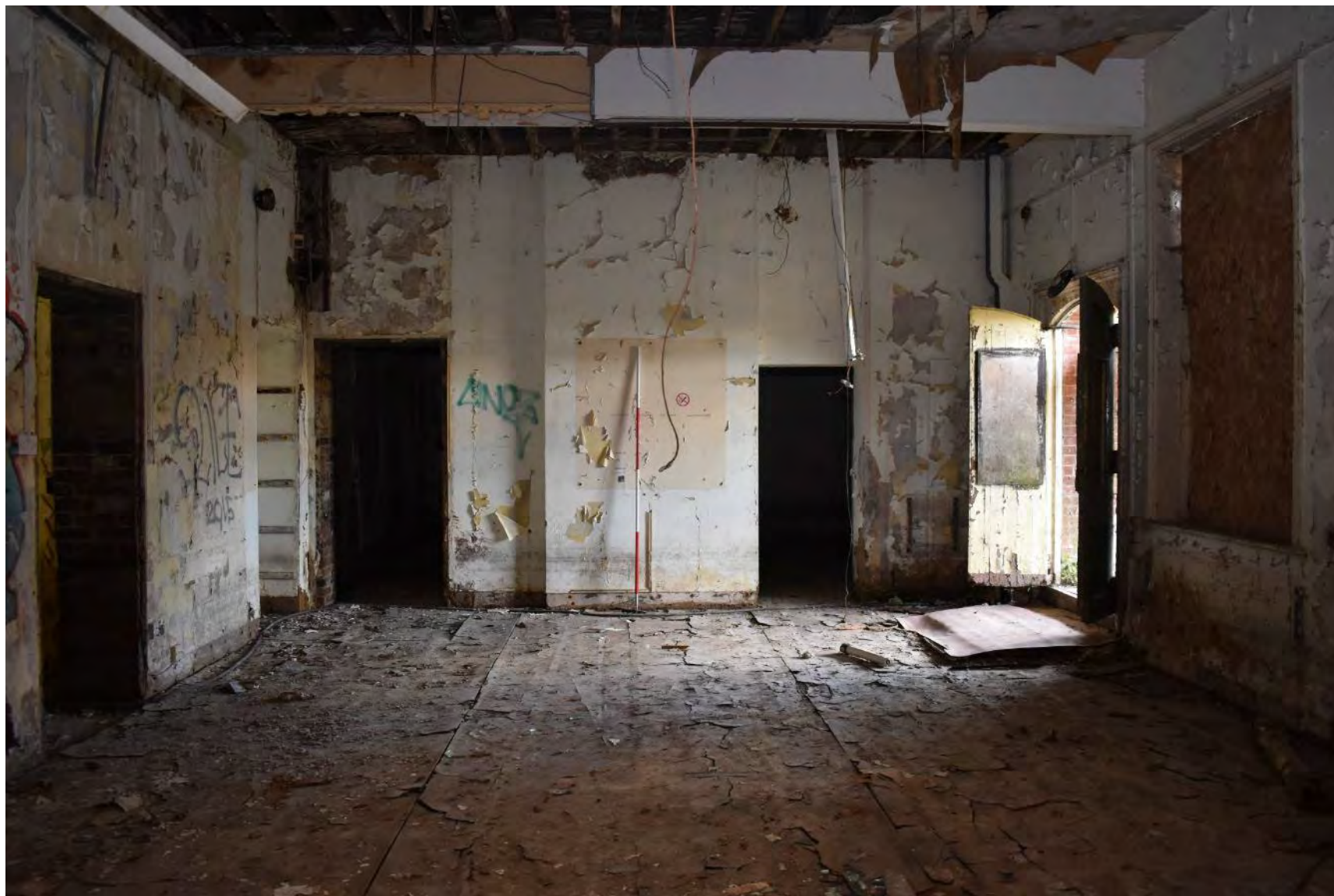
Plate 66: Room D (August 2021 facing W)
