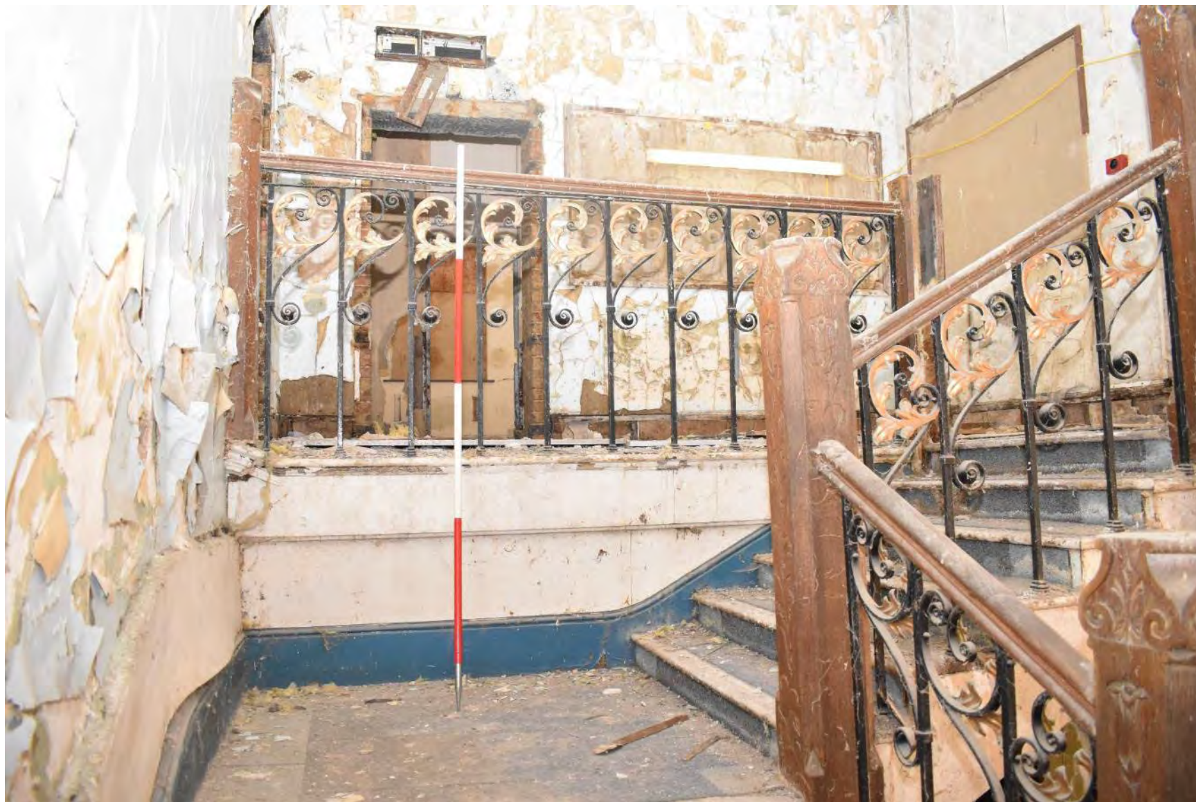
Plate 102: Ground floor to first floor staircase (August 2021 facing N)
