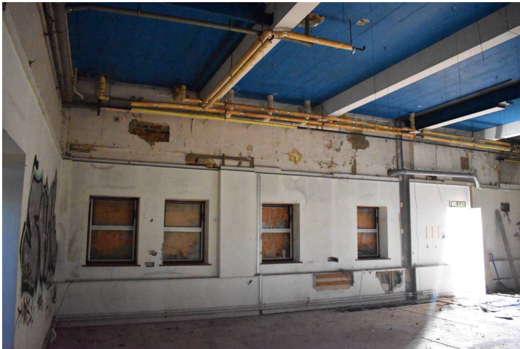
Plate 132: Depot Ground Floor (December 2022 facing SE)
