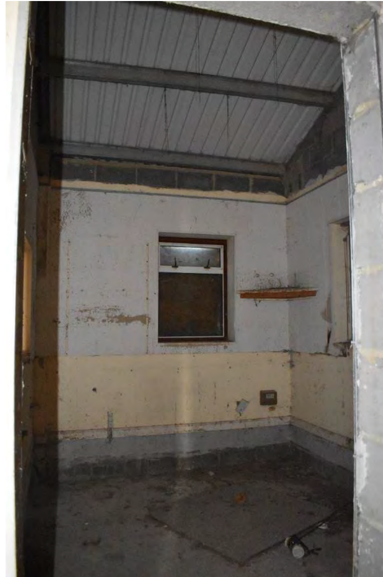
Plate 124: Depot upper floor modern extension (December 2022 facing NW)
