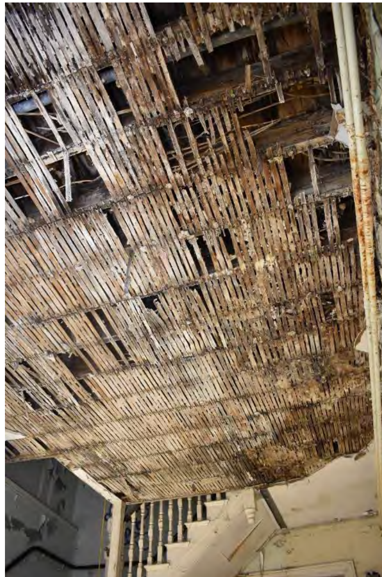
Plate 65: Room C ceiling (August 2021)
