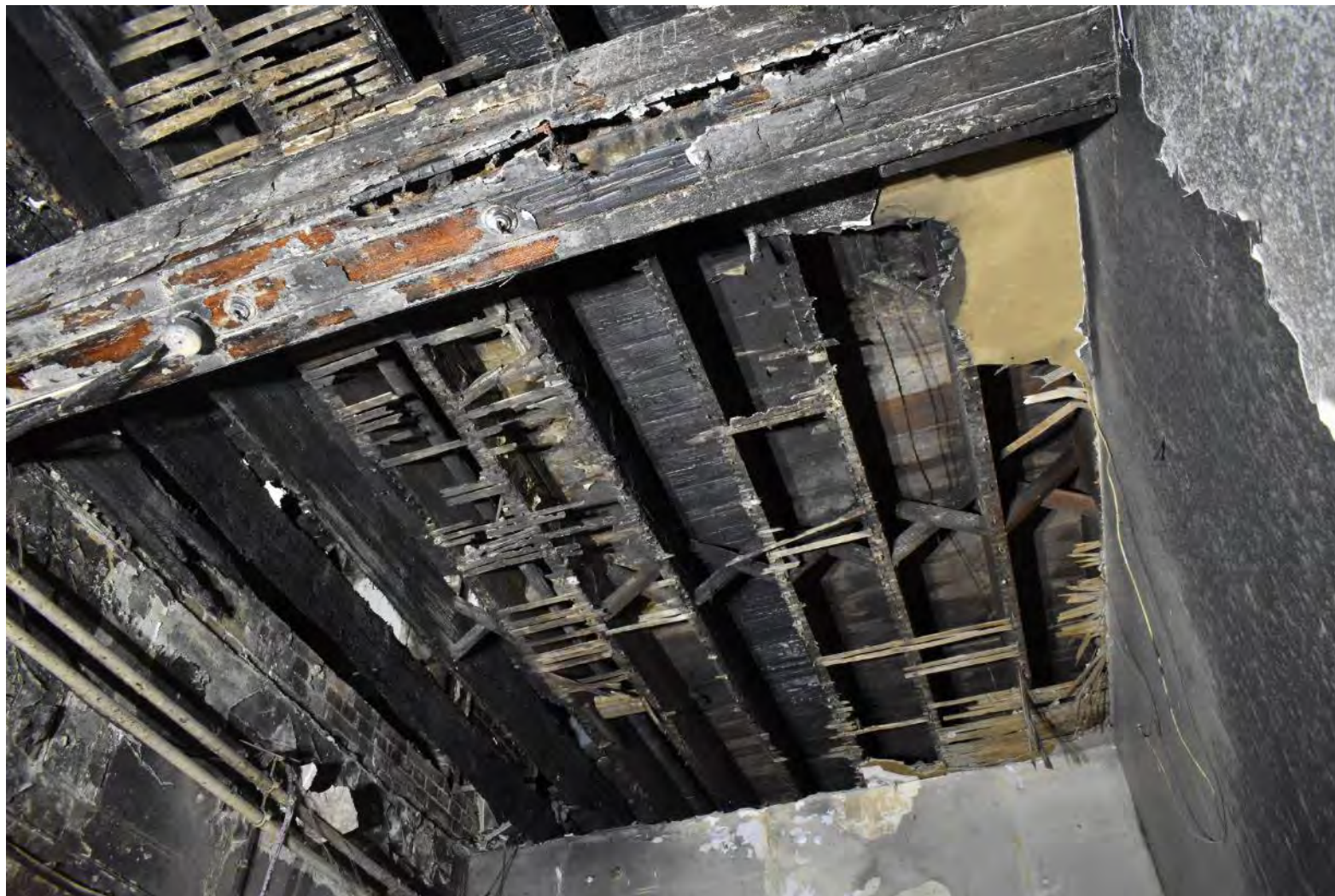
Plate 136: Main Office, Basement, Room H ceiling
