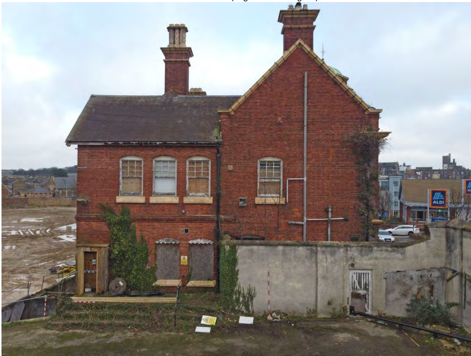
Plate 18: Front View (August 2021 facing SW).
