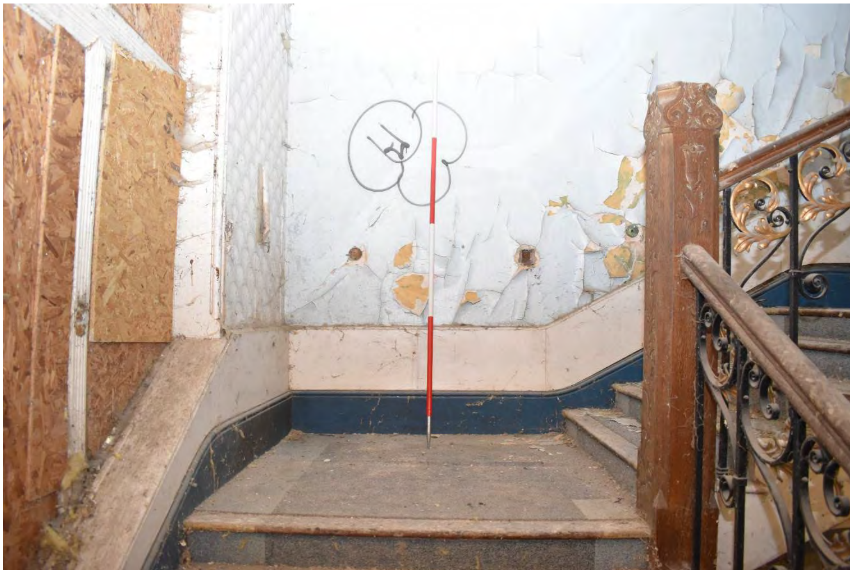
Plate 100: Ground floor to first floor staircase (August 2021 facing W)
