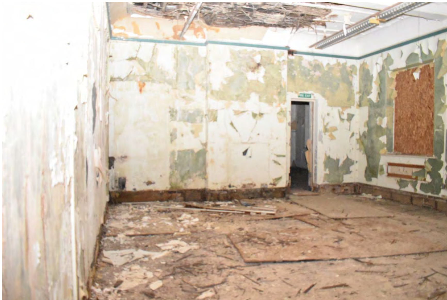
Plate 97: Room N (August 2021 facing WNW)
