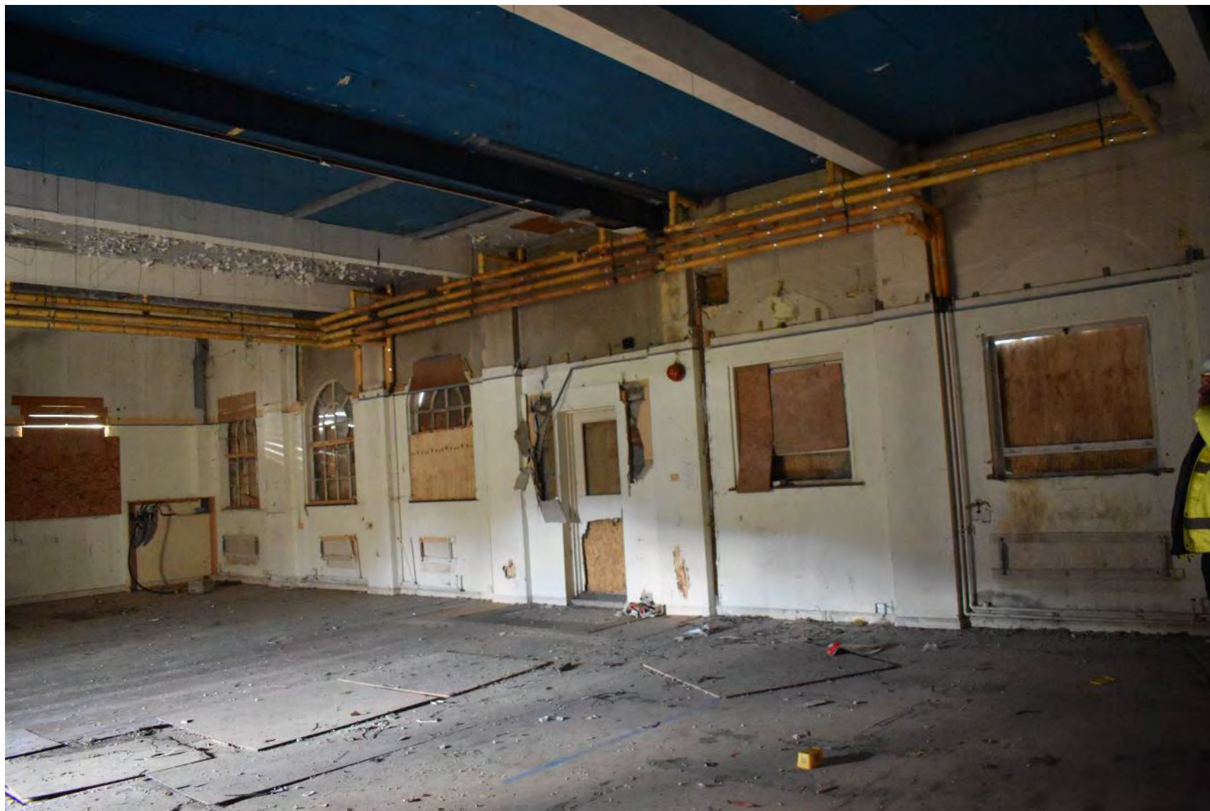
Plate 126: Depot Ground Floor (December 2022 facing SW )
