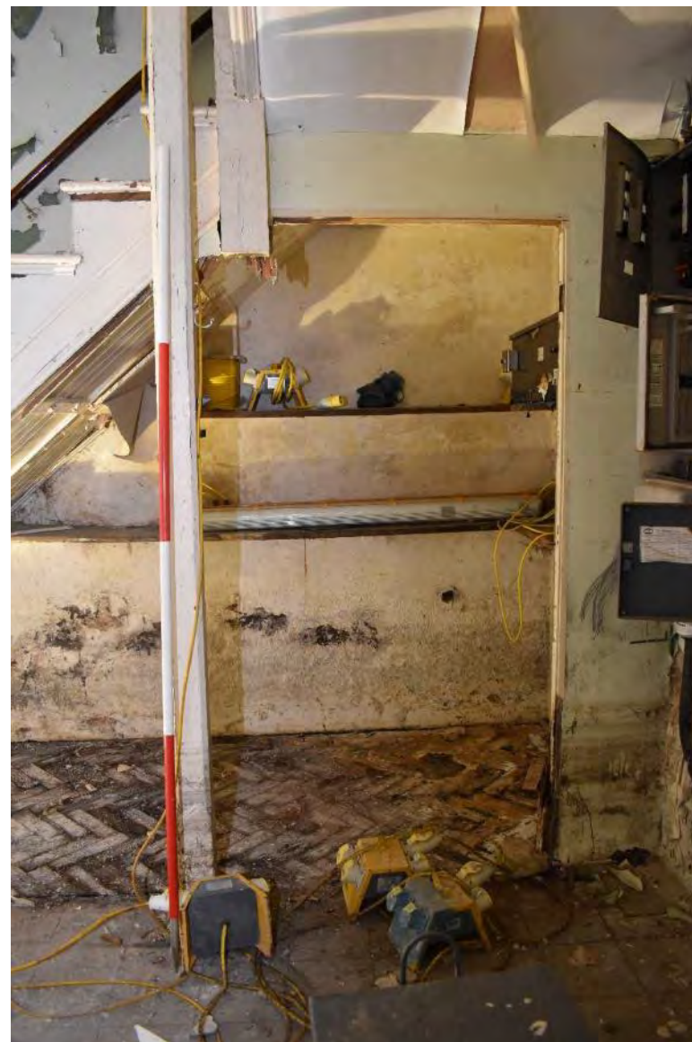
Plate 63: Room C (August 2021 facing E)
