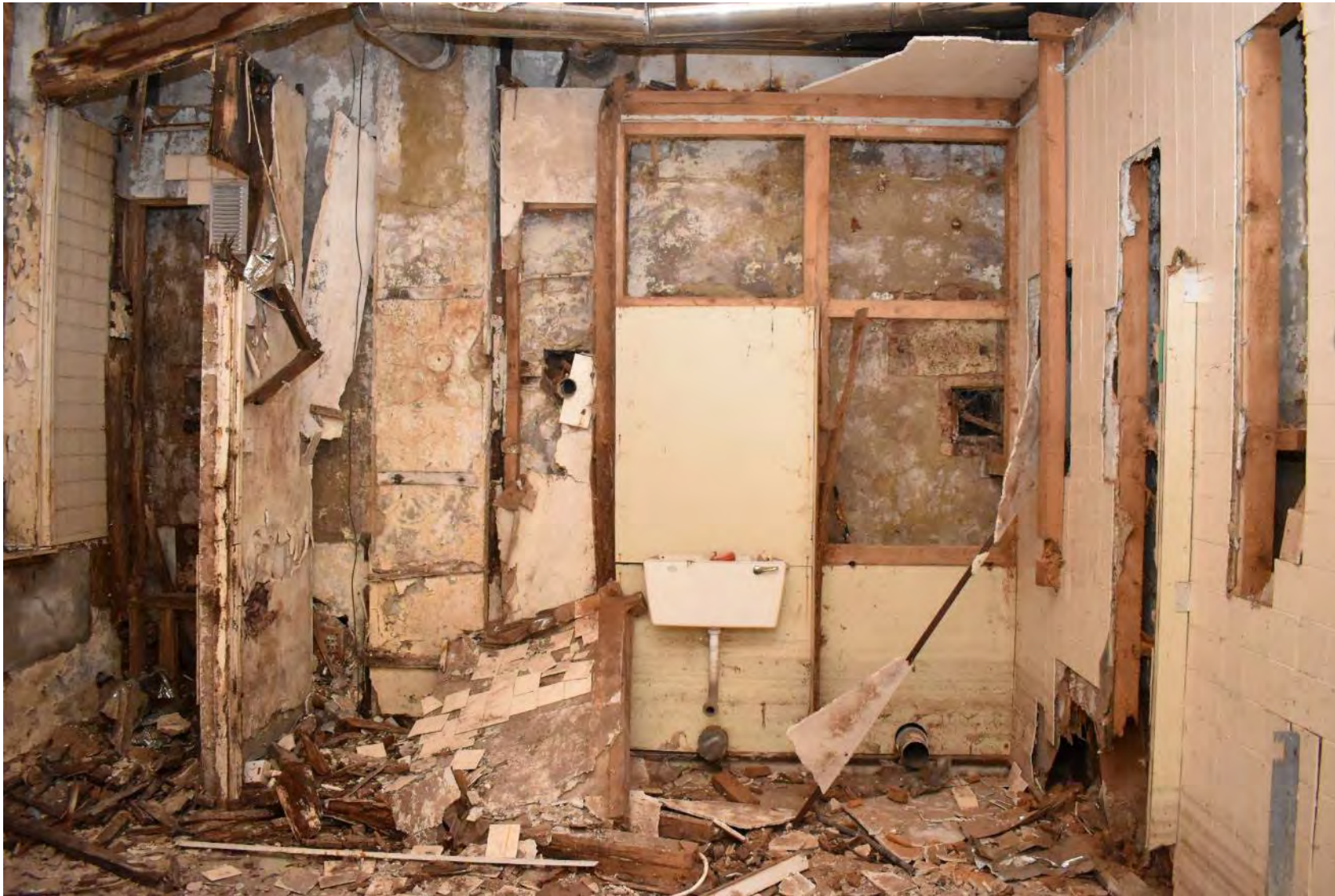
Plate 52: Room A (August 2021 facing SW)
