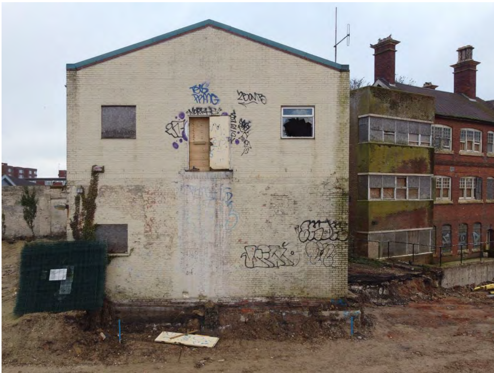
Plate 41: Adjoining building, northern side (December 2020)
