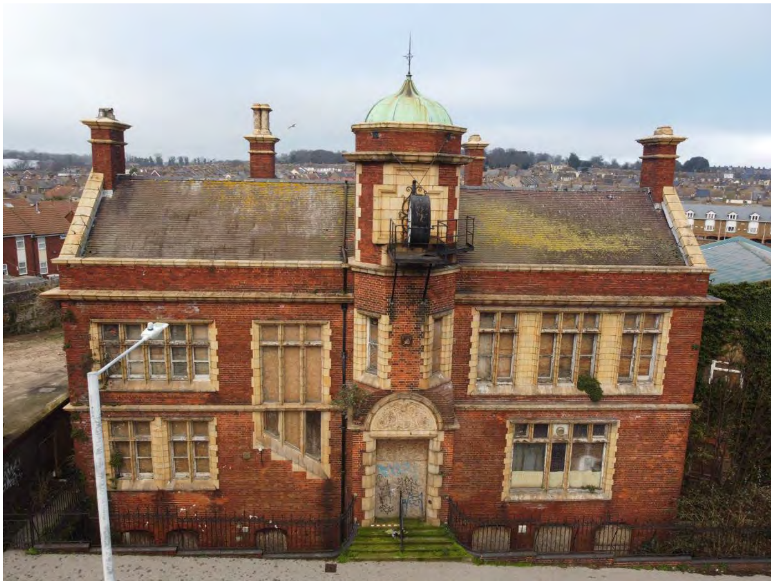
Plate 27: Roof view at the front (December 2020 facing SE).
