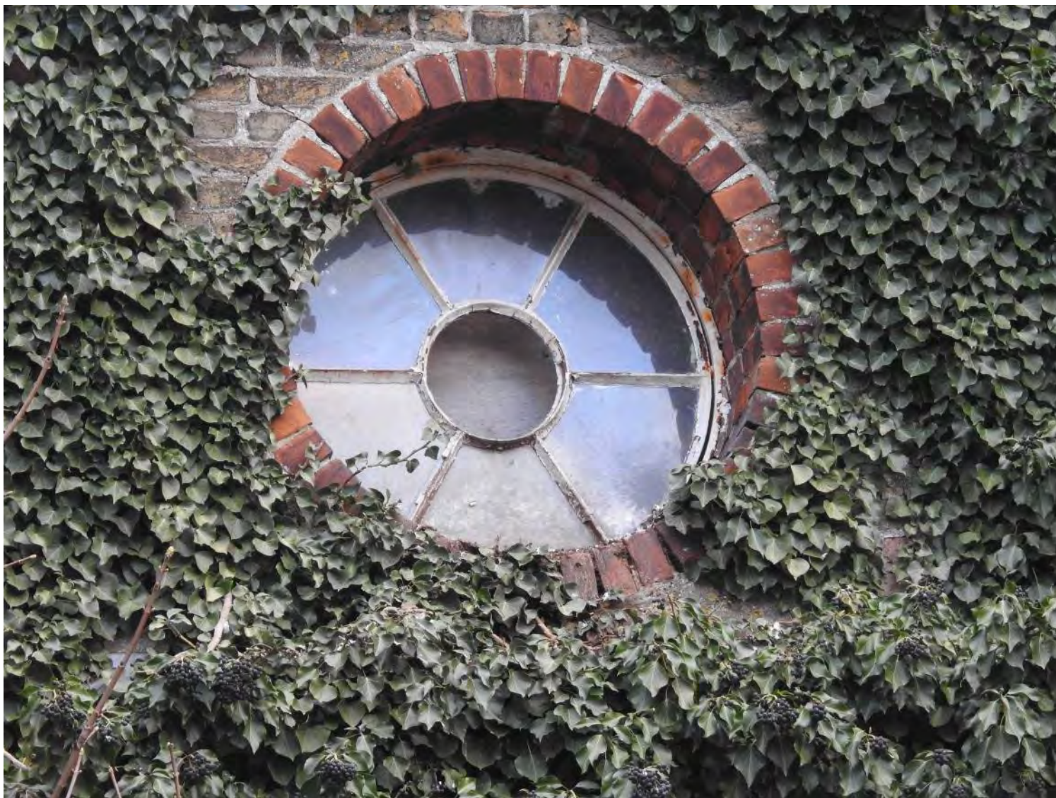
Plate 42: Window details on adjoining building southern side (December 2020)
