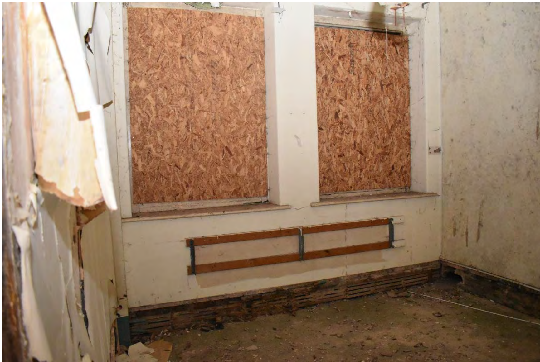
Plate 93: Room L (August 2021 facing NW)
