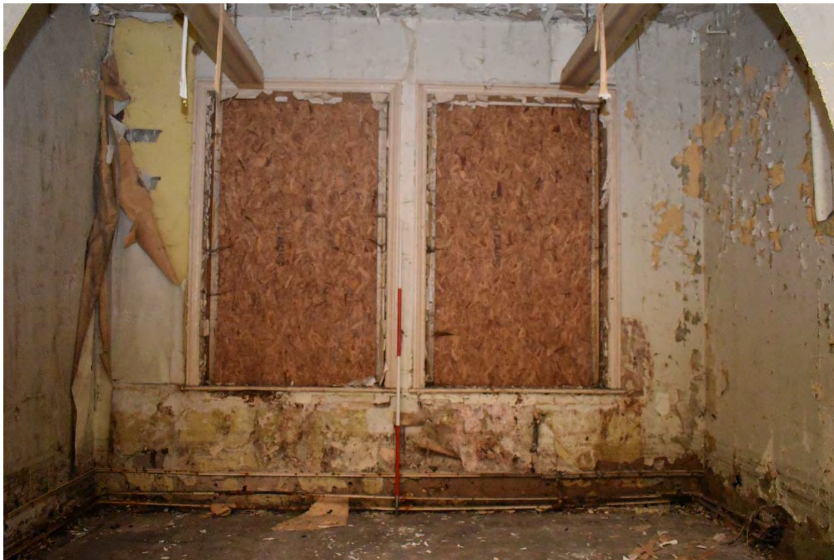
Plate 73: Room E (August 2021 facing N)
