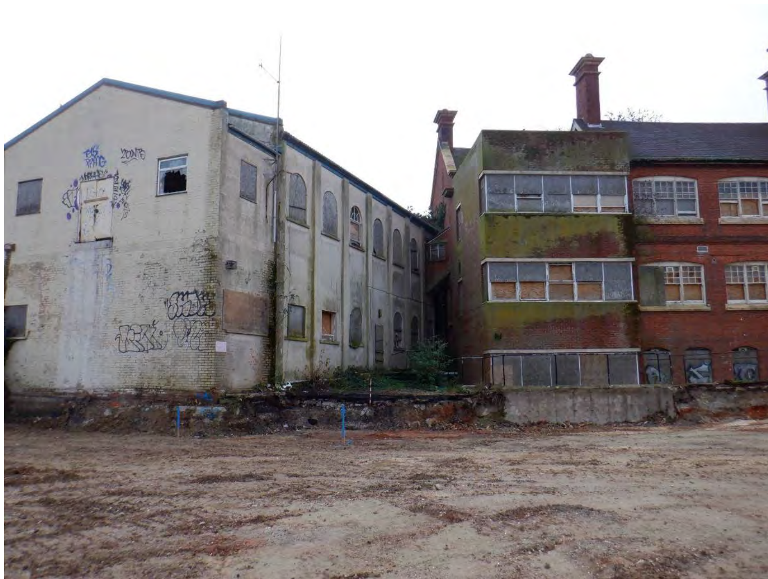
Plate 21: View of the join between the buildings (December 2020 facing NNW)
