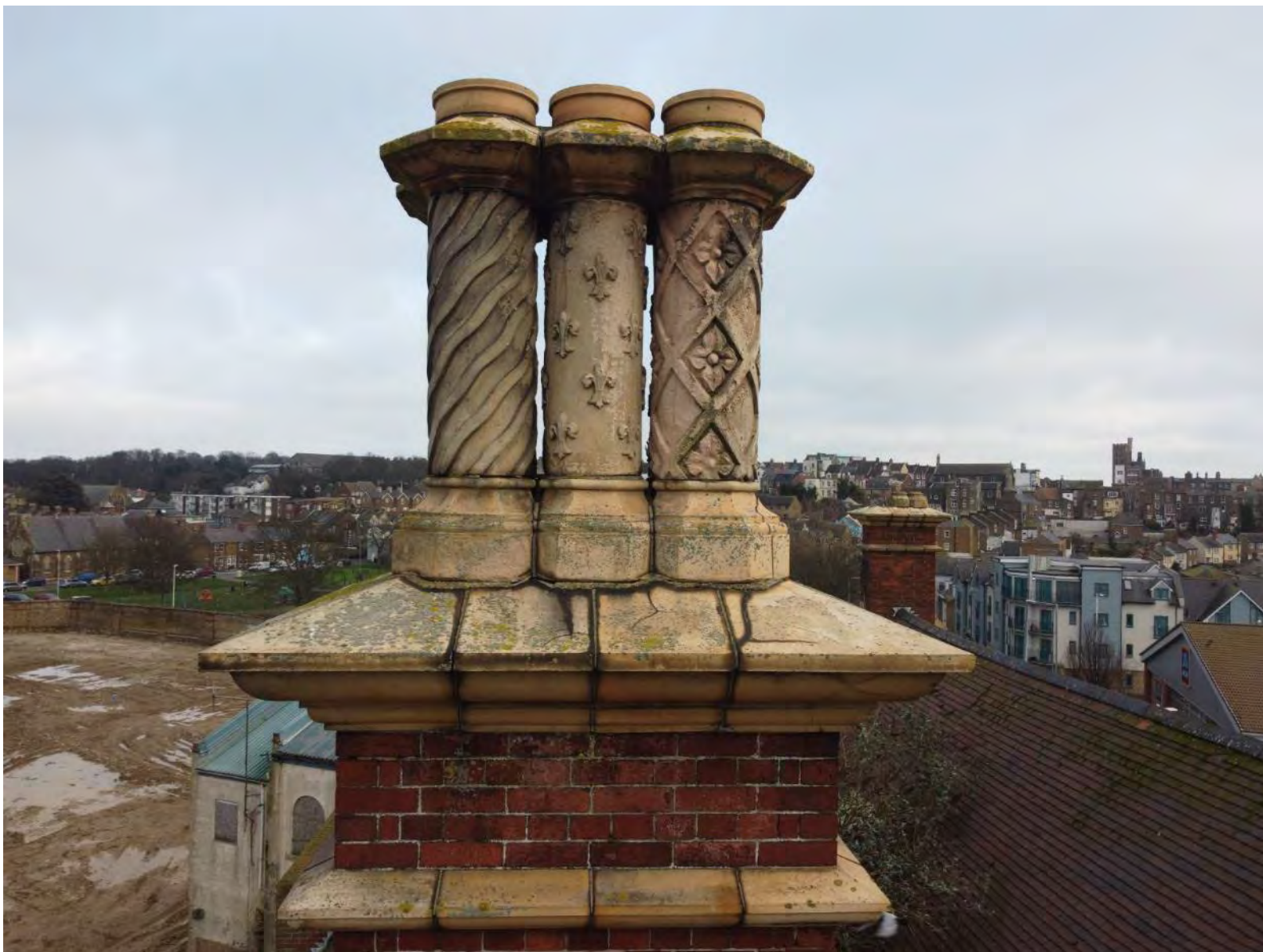
Plate 23: Close up of the Chimneys western side (December 2020)
