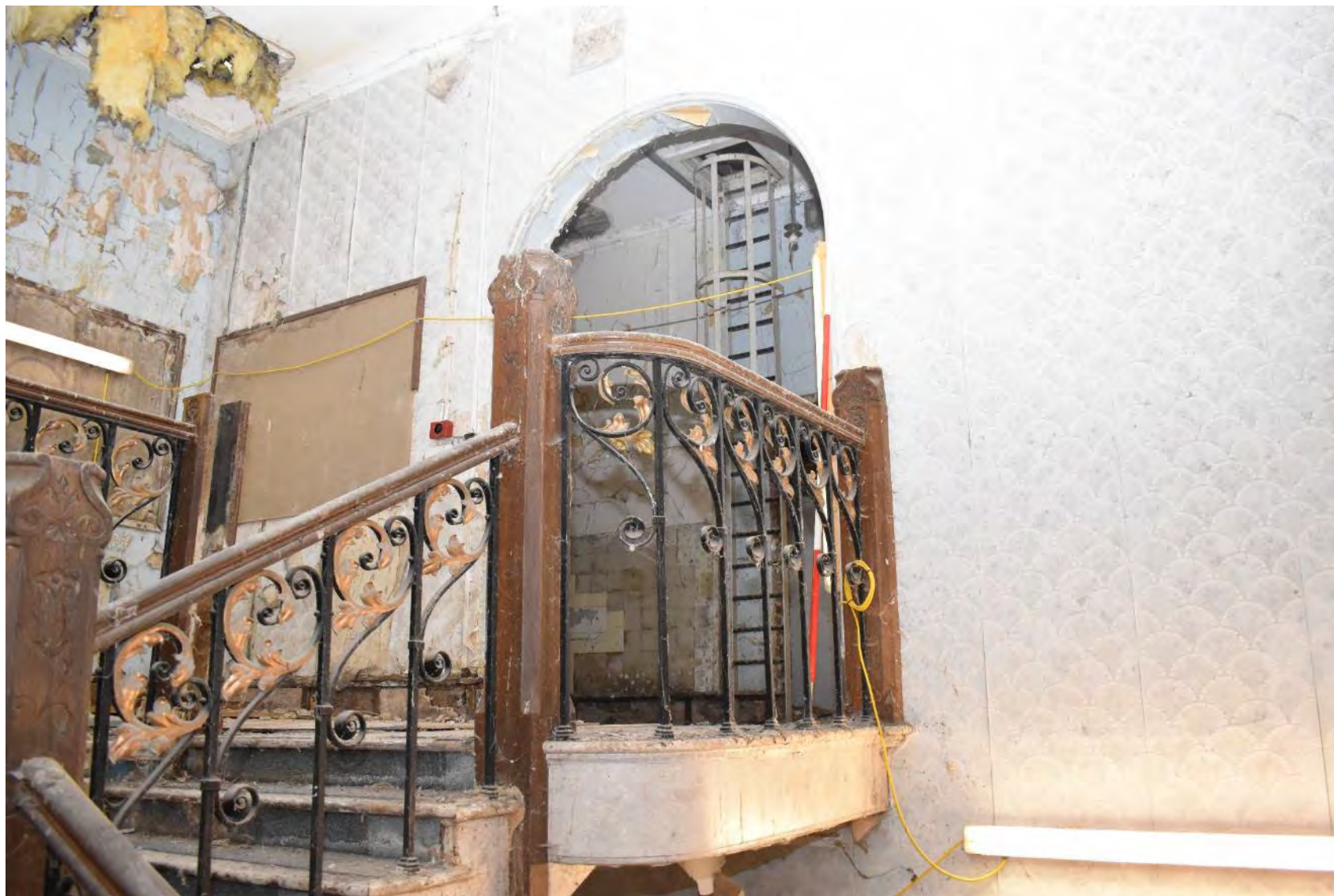
Plate 103: Ground floor to first floor staircase (August 2021 facing NE)
