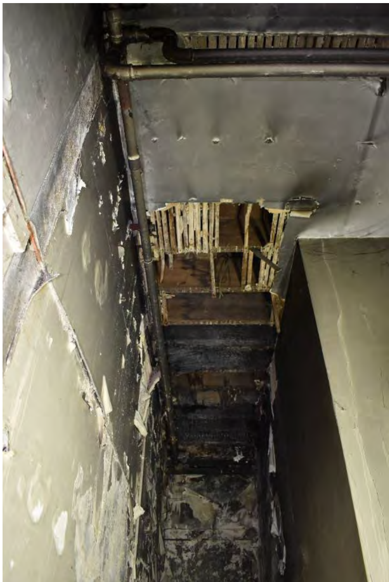
Plate 139: Main Office, Room G corridor ceiling
