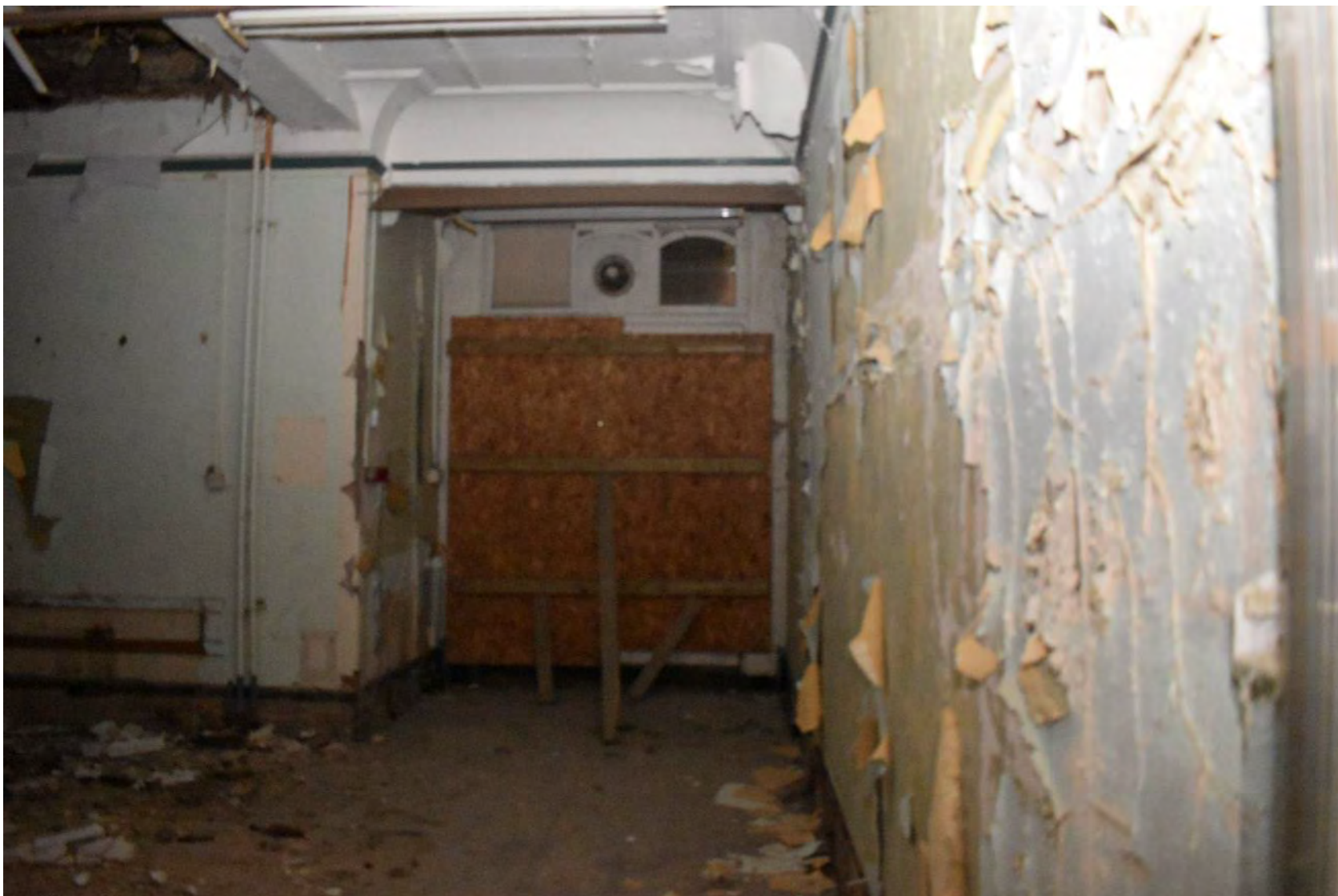
Plate 96: Room M entrance area (August 2021 facing S)
