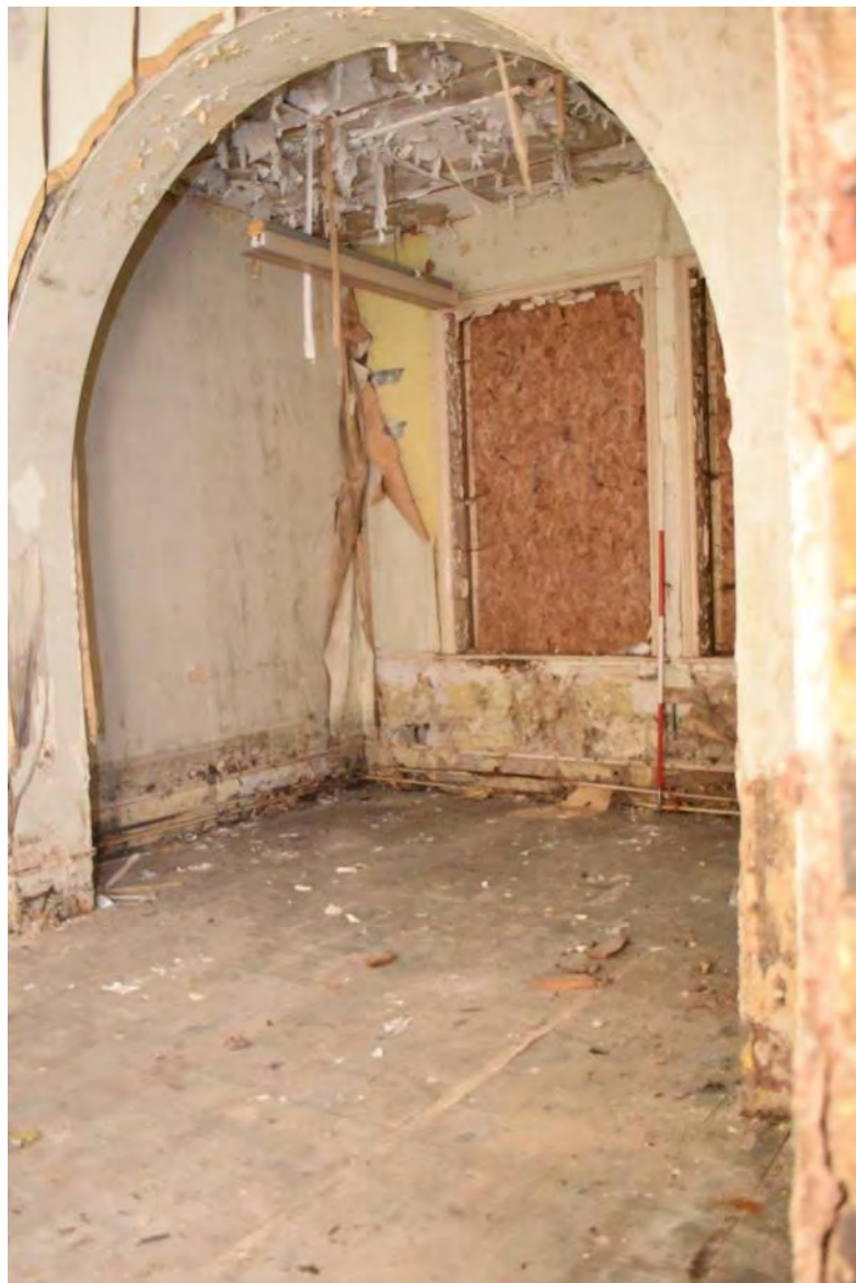
Plate 71: Room E (August 2021 facing NW)
