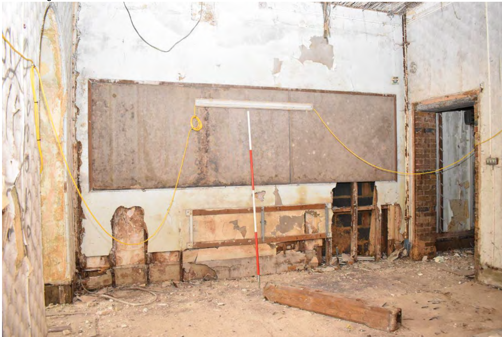
Plate 87: Room I - Ground floor lobby (August 2021 facing NNE)
