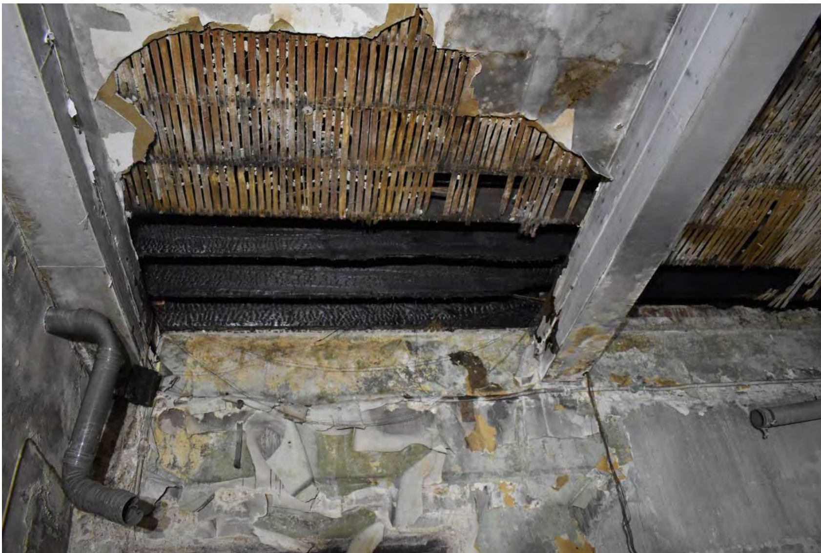
Plate 138: Main Office, Basement, Room G ceiling
