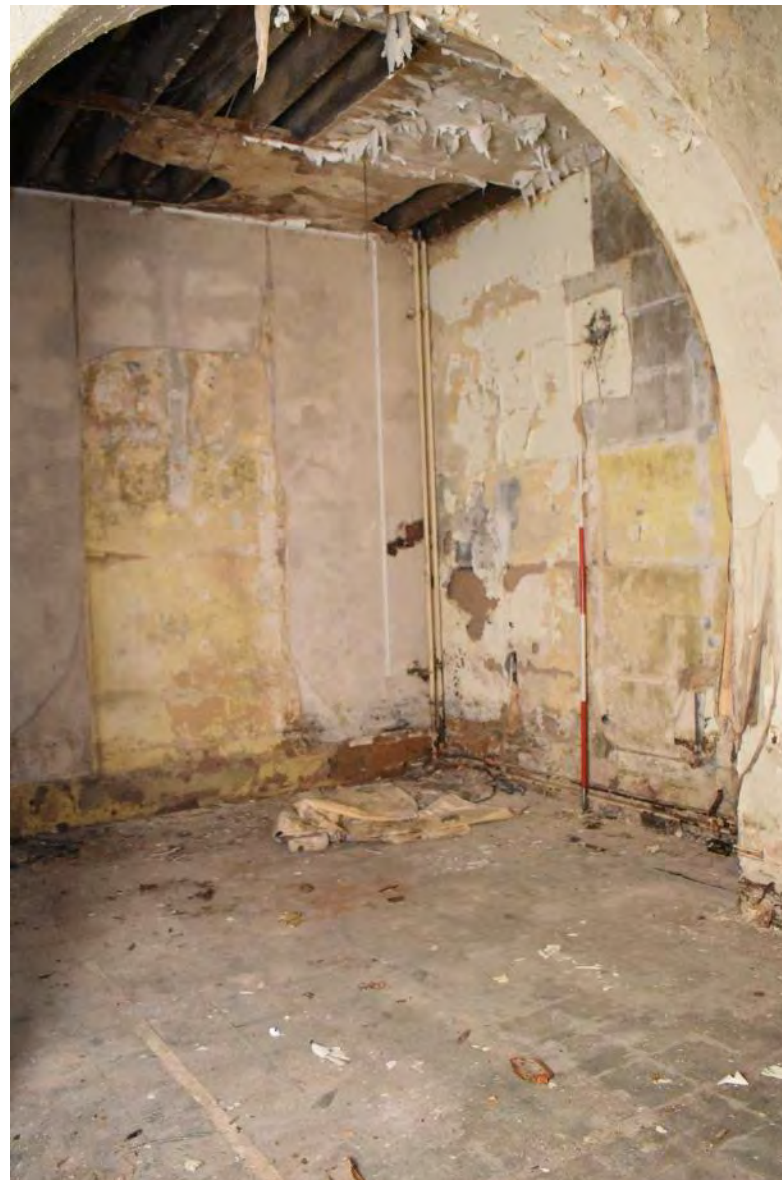
Plate 72: Room E (August 2021 facing SW)
