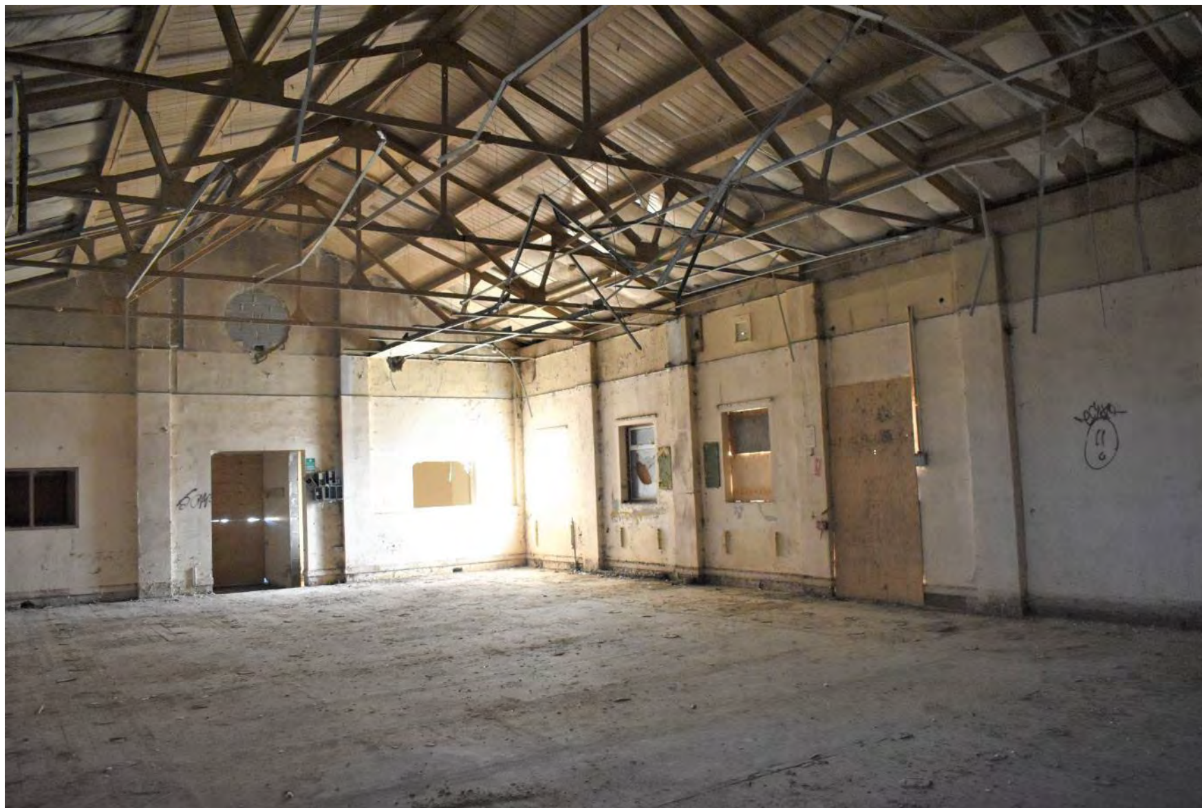
Plate 121: Depot Upper Floor (December 2022 facing NE)
