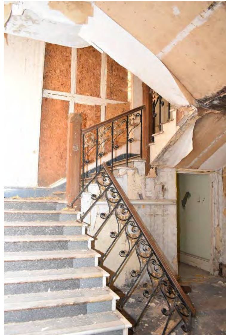
Plate 89: Ground Floor staircase (August 2021 facing SW)
