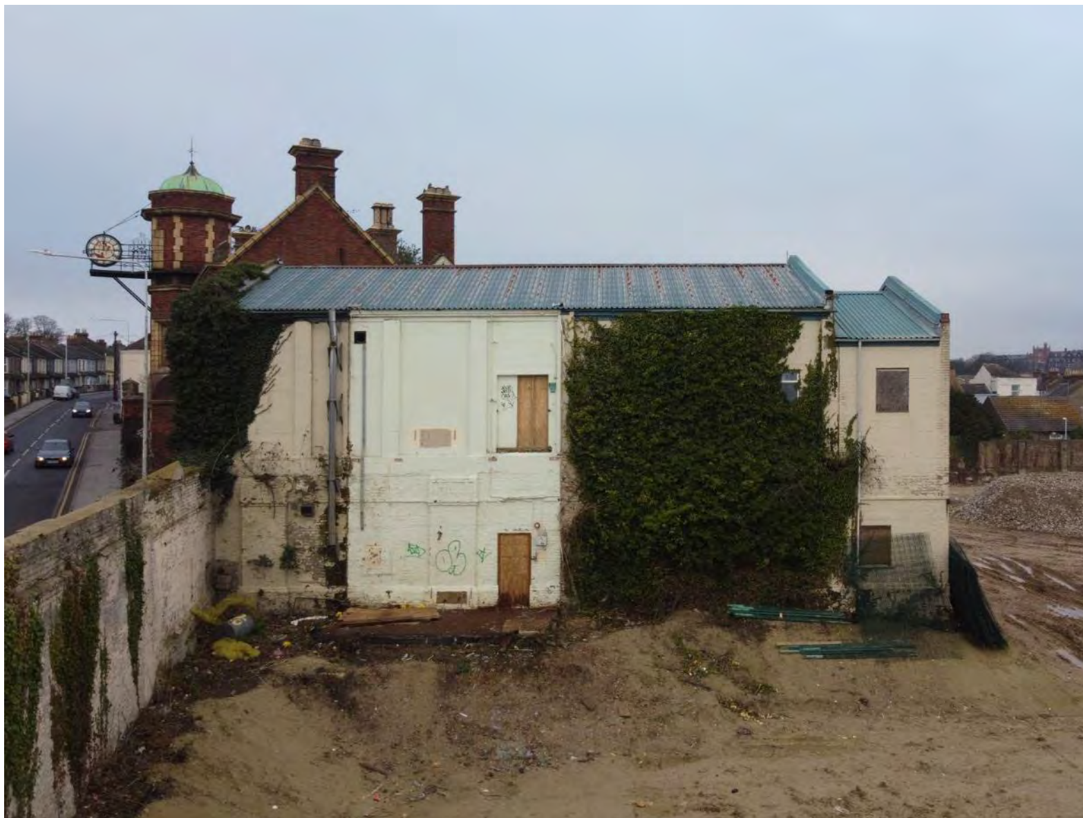
Plate 39: Adjoining building eastern side (December 2020 facing N)
