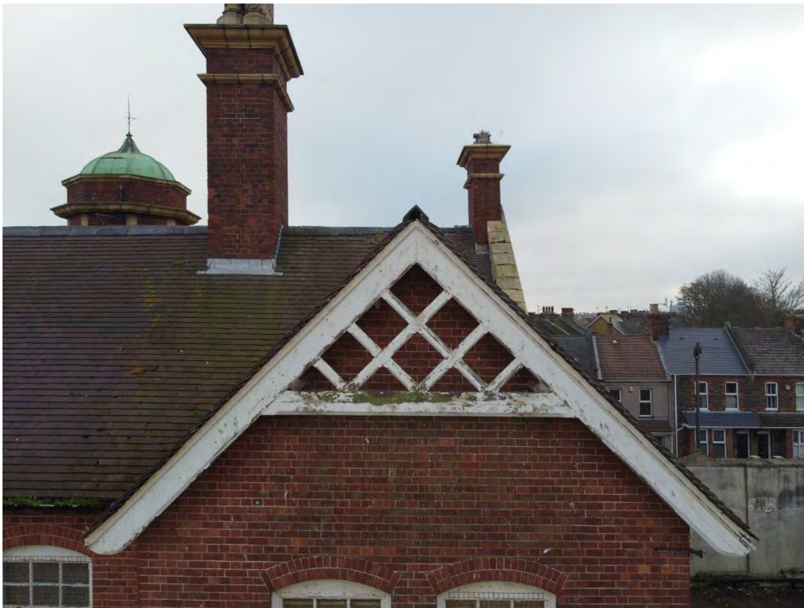
Plate 36: Gable end detail at the rear (December 2020 facing SE).
