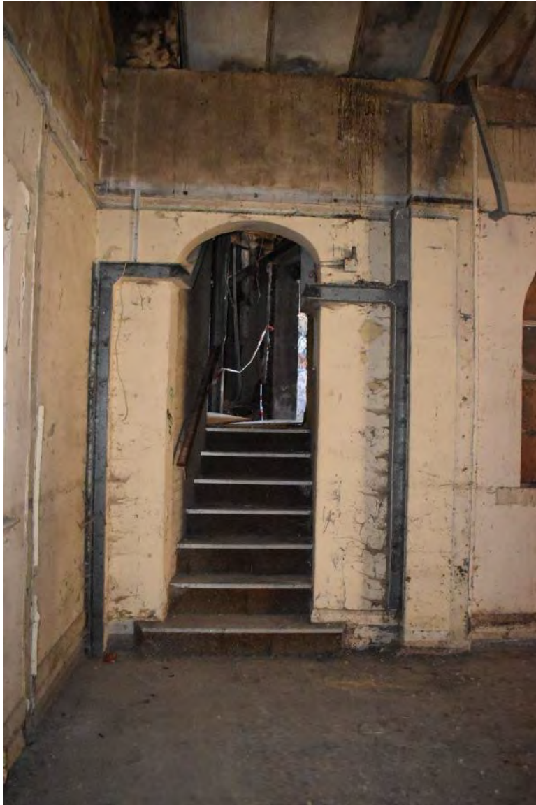
Plate 123: Upper Floor Stair to main offices from Depot (December 2022)
