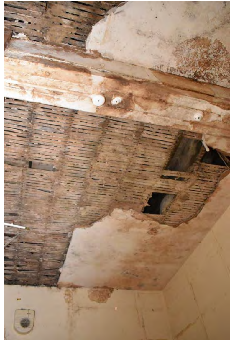
Plate 85: Room H ceiling (August 2021)
