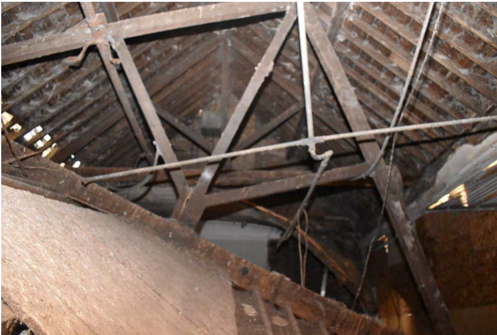
Plate 114: Roof above Room S (August 2021)
