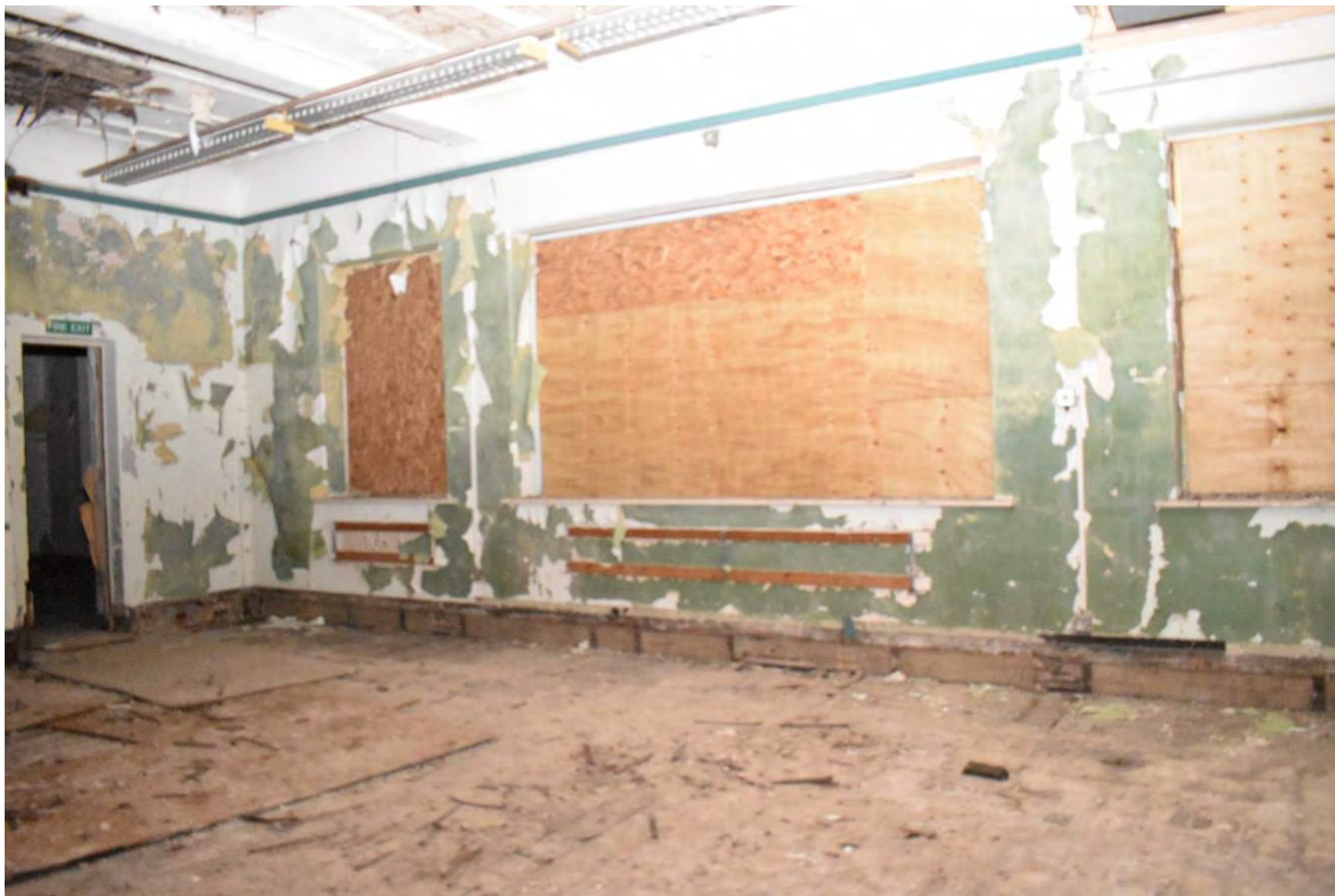
Plate 98: Room N (August 2021 facing NW)
