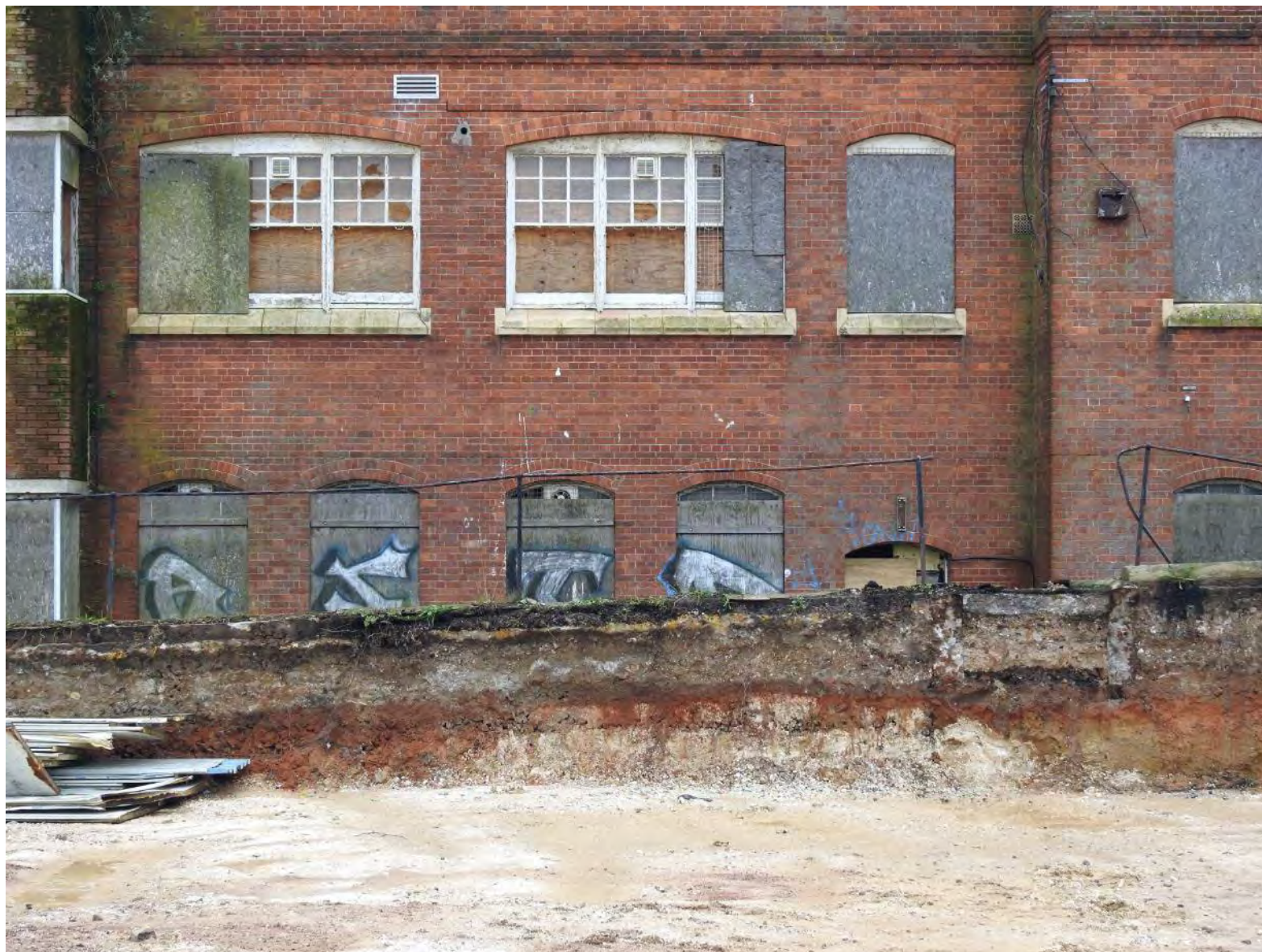
Plate 37: Window detail at the rear of the office building (December 2020)
