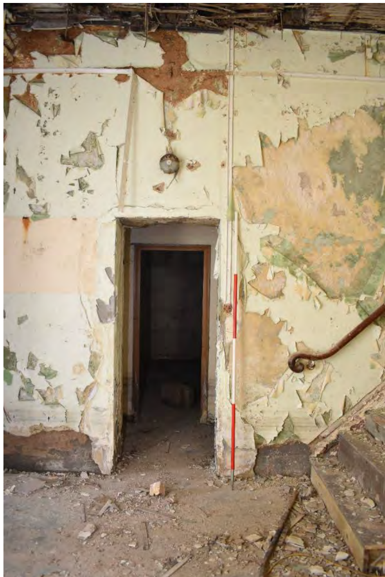
Plate 64: Room C into Room H (August 2021 facing E)
