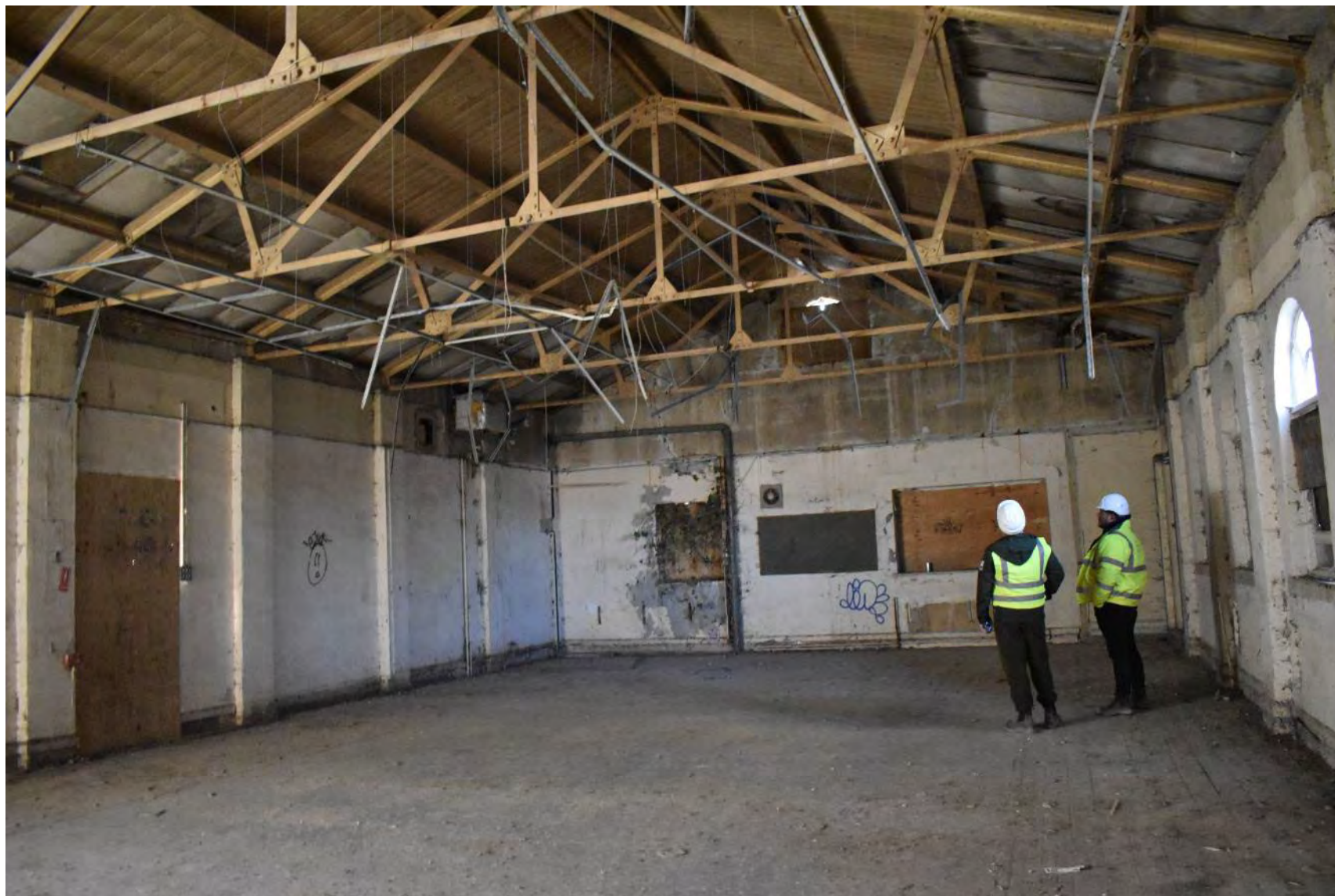
Plate 122: Depot Upper Floor (December 2022 facing S)
