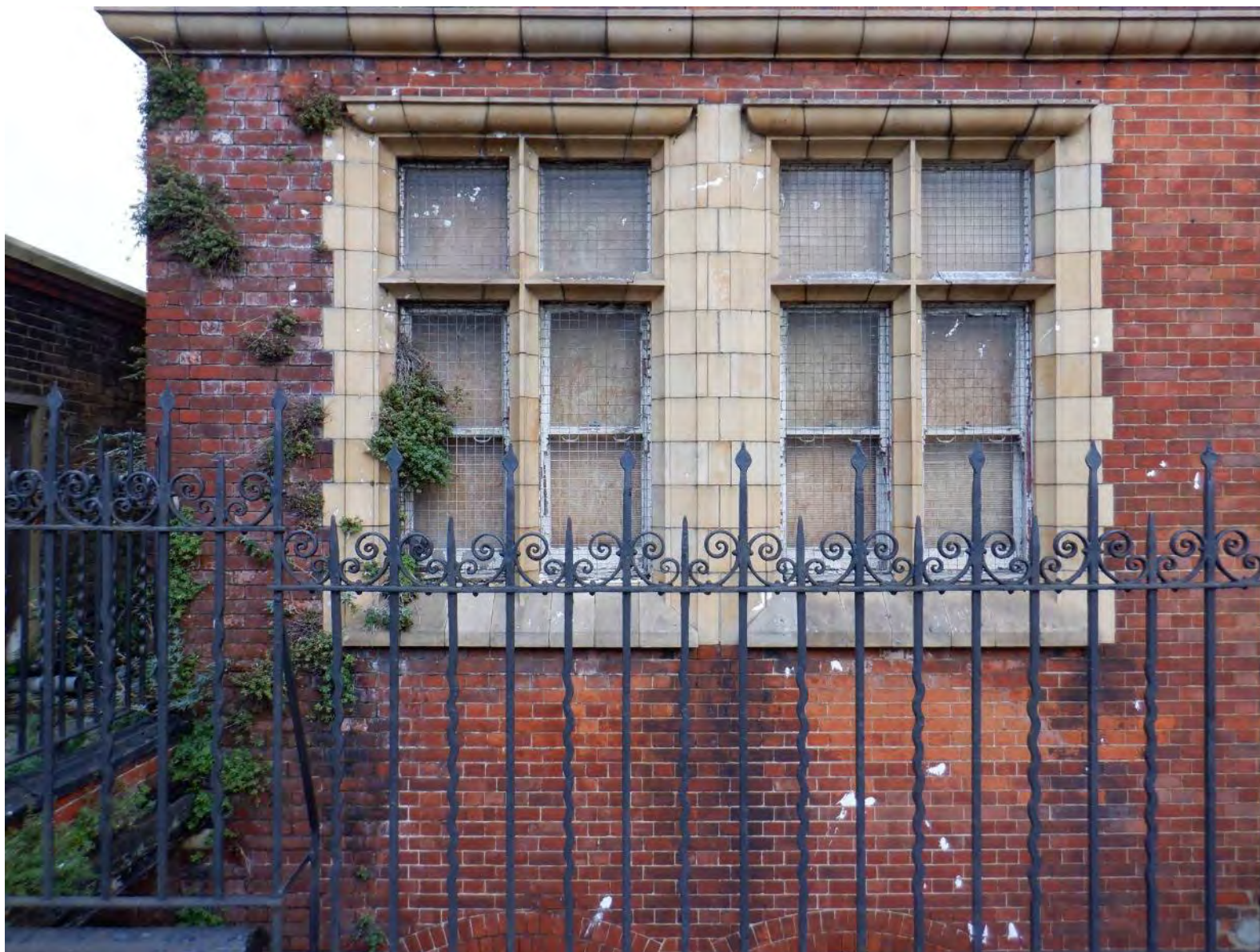
Plate 34: Detail of front windows western side of the ground floor (December 2020).
