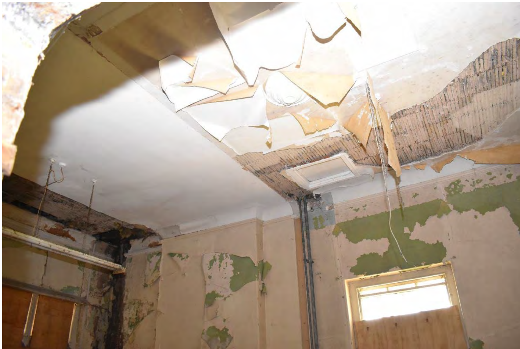
Plate 106: Room O ceiling (August 2021)
