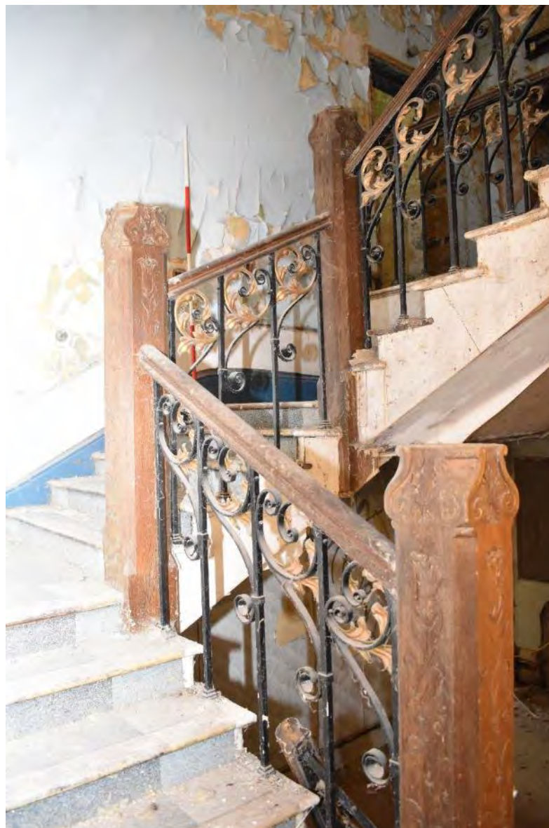
Plate 101: Ground floor to first floor staircase (August 2021 facing NW)
