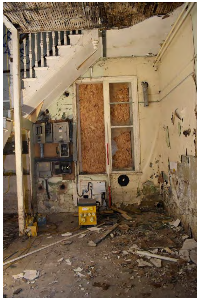
Plate 59: Room C (August 2021 facing N)
