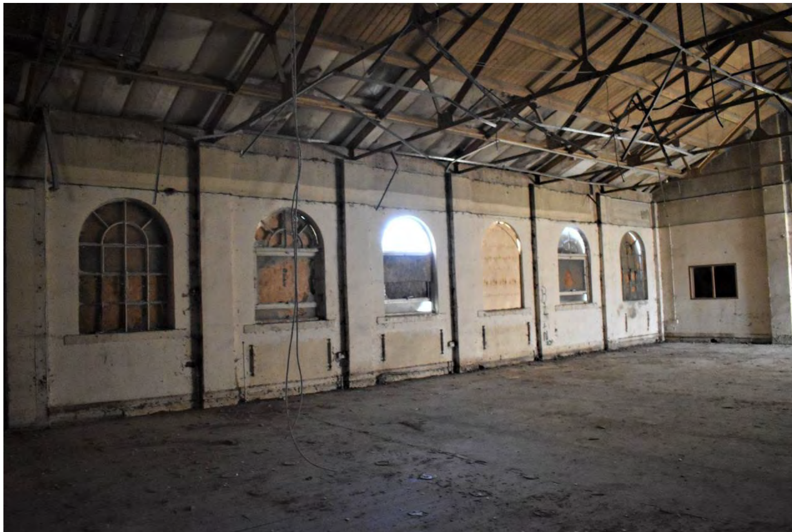
Plate 120: Depot Upper Floor (December 2022 facing NNE)
