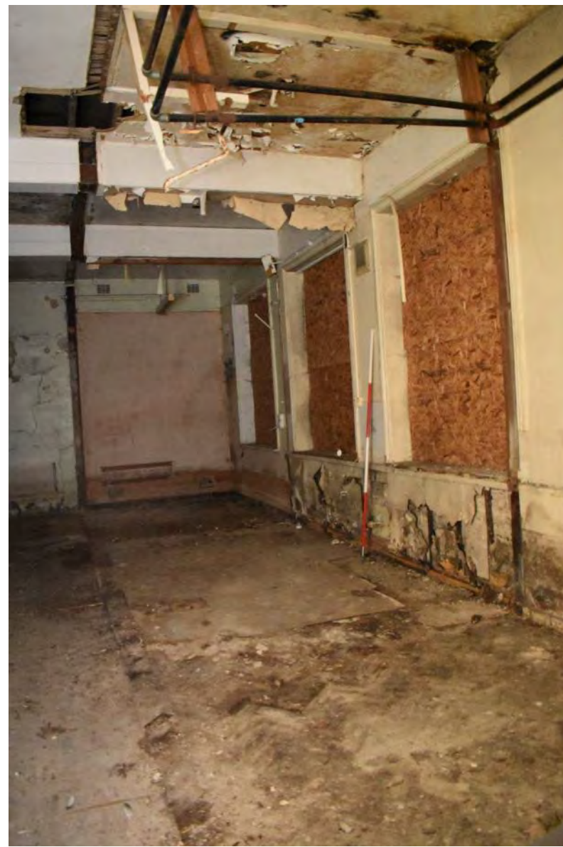
Plate 81: Room G (August 2021 facing SE)
