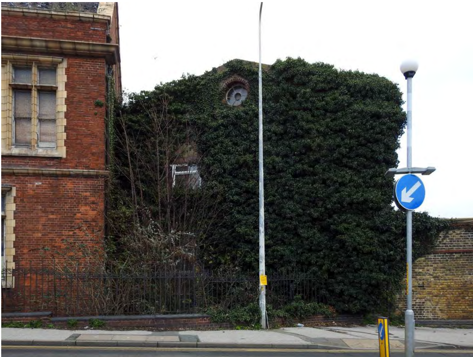
Plate 40: Adjoining building from Boundary Road, southern side (December 2020)
