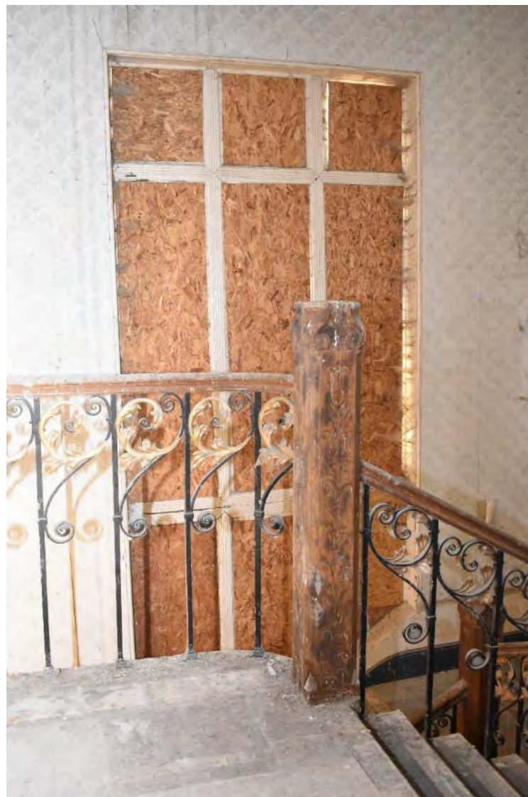
Plate 119: Staircase window (August 2021 facing SW)
