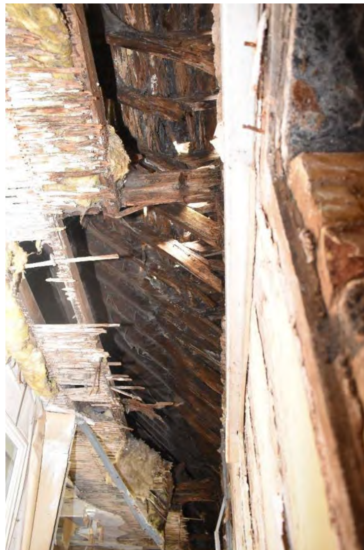
Plate 108: Room P ceiling (August 2021)
