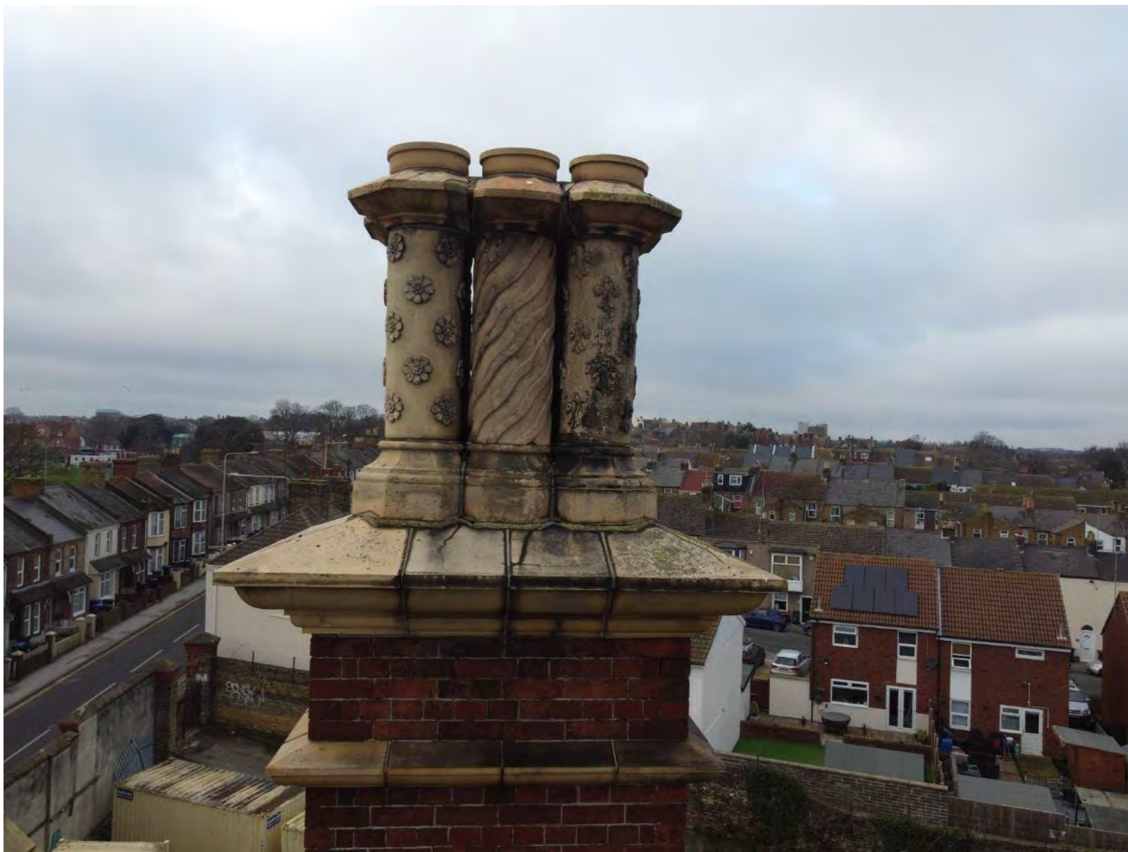
Plate 24: Close up of Chimneys on eastern side ( December 2020)
