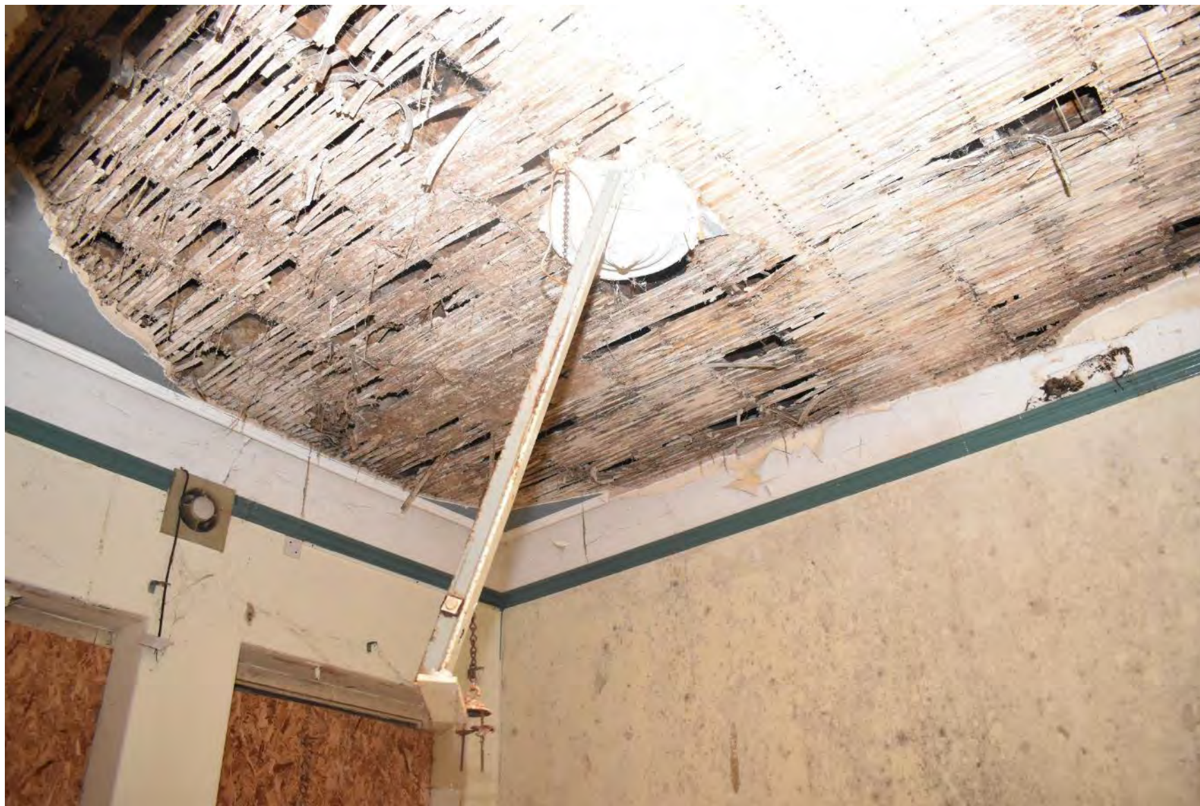
Plate 94: Room L ceiling (August 2021)
