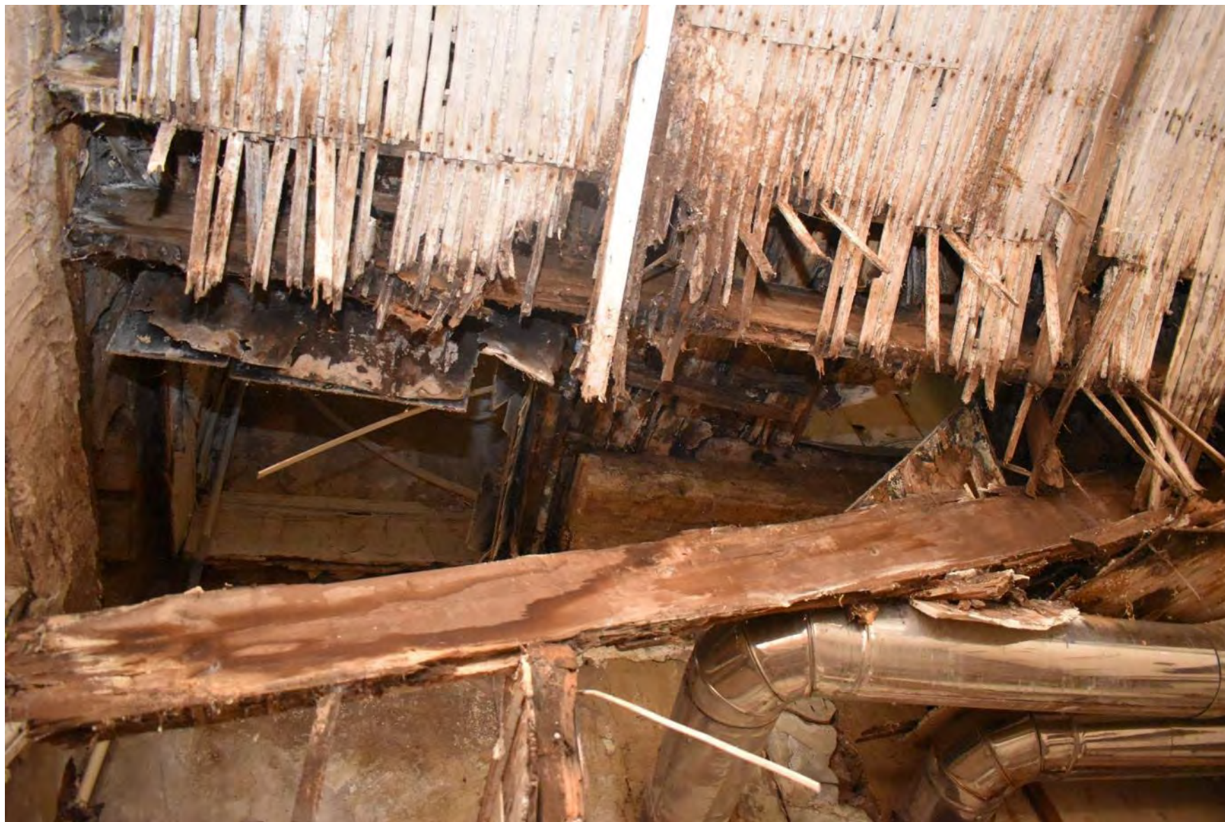
Plate 56: Room A – ceiling (August 2021)
