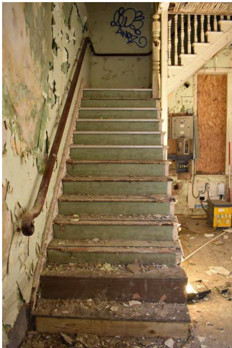
Plate 62: Room C (August 2021 facing N)
