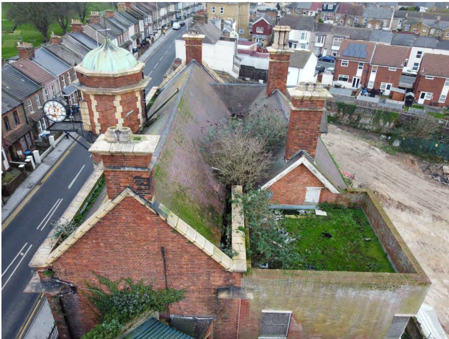
Plate 26: Roof view at the eastern end (December 2020)
