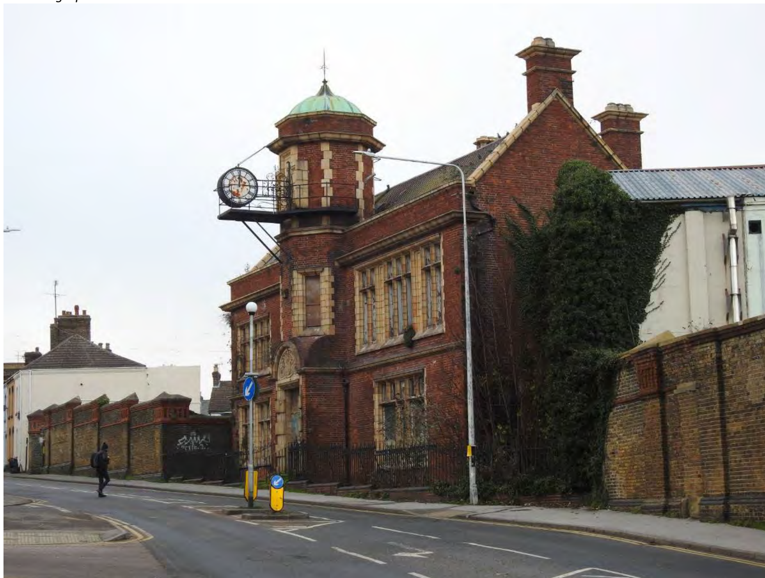
Plate 17: View of the office from Boundary Road (August 2021 facing SSW)
