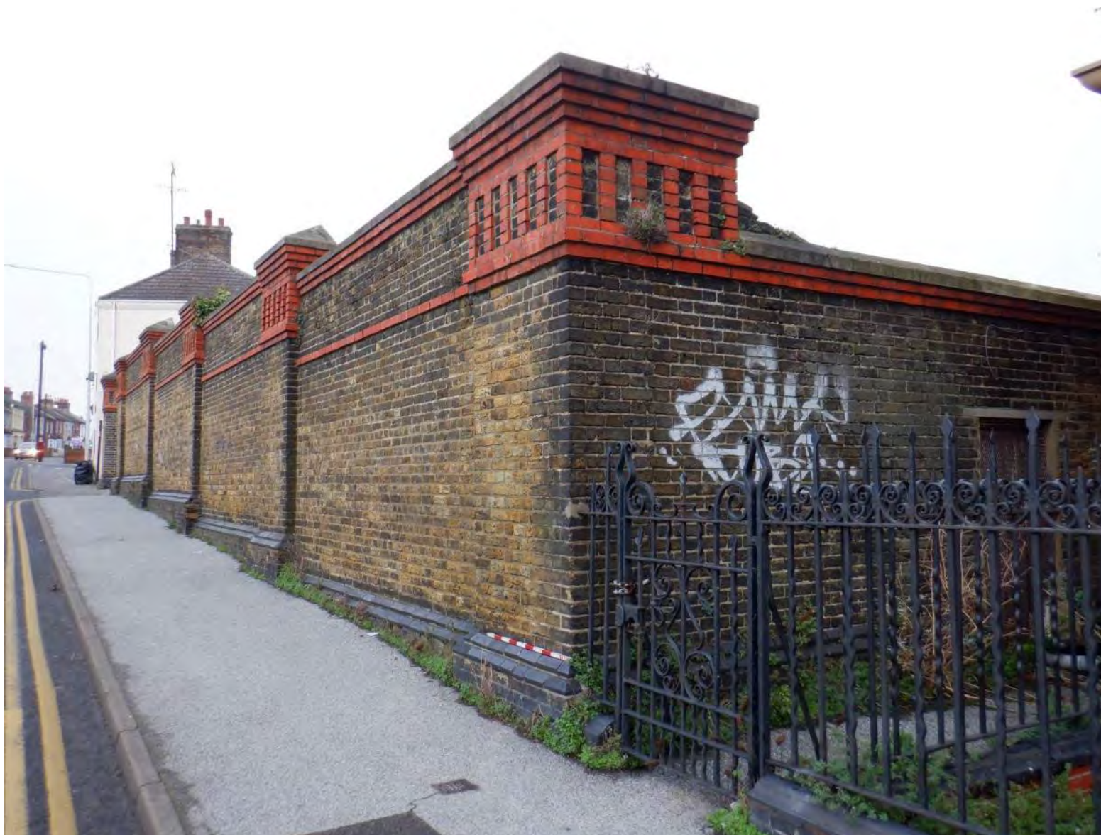
Plate 46: Corner of wall by south western corner of the main building, scale 1m (August 2021 facing NW)
